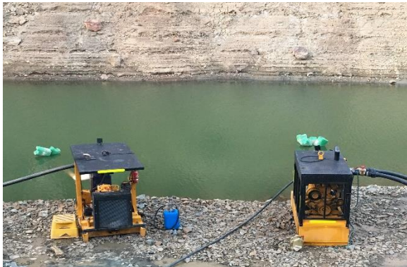
Photo 1. Pit dewatering pumps in action.
