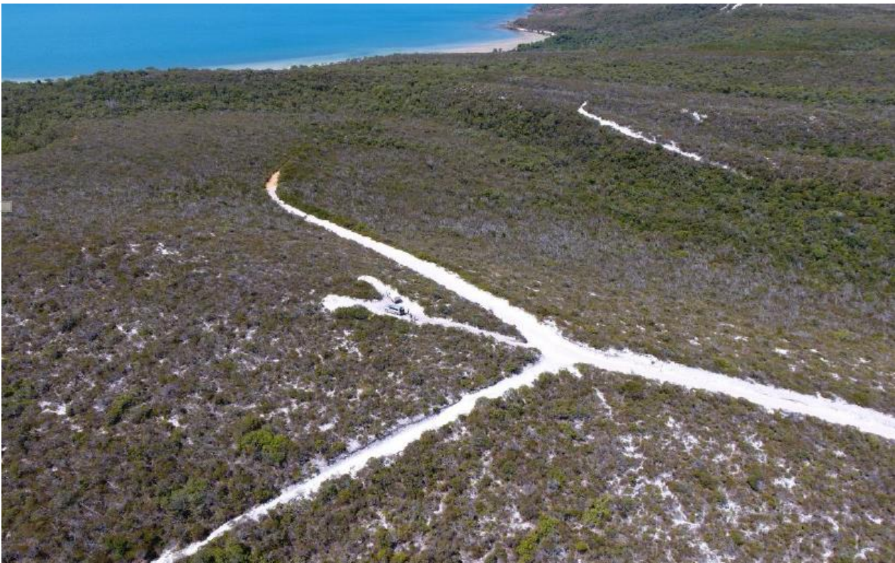
Aerial photo of tracks to be drilled at the Cape Flattery Silica Sand Project and the Port of Cape Flattery
