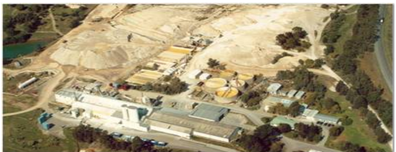
Figure 2: Pittong processing plant facilities
