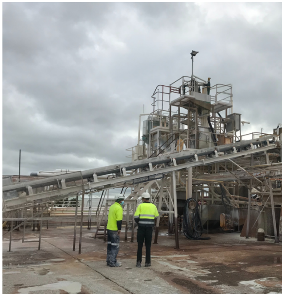
Figure 3: Pittong processing plant facilities
