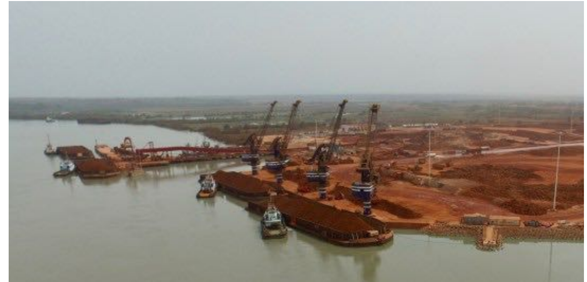
Image 3 – Katougouma Export Terminal. Currently handling c 18Mtpa Bauxite ore from SMB. (Not Assets of Lindian Resources)
