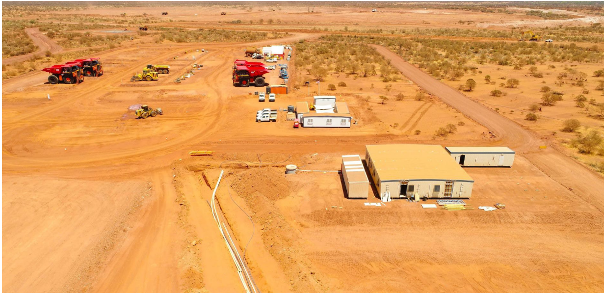
Establishment of mining contractor
