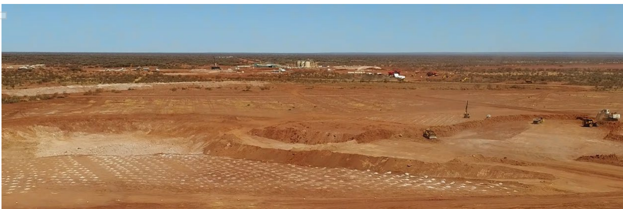
Drill & blast drilling (foreground) and grade control drilled area (middle)
