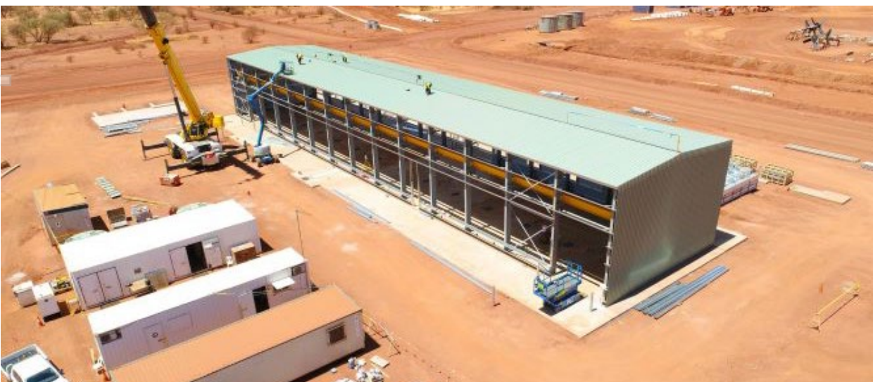
Power station construction
