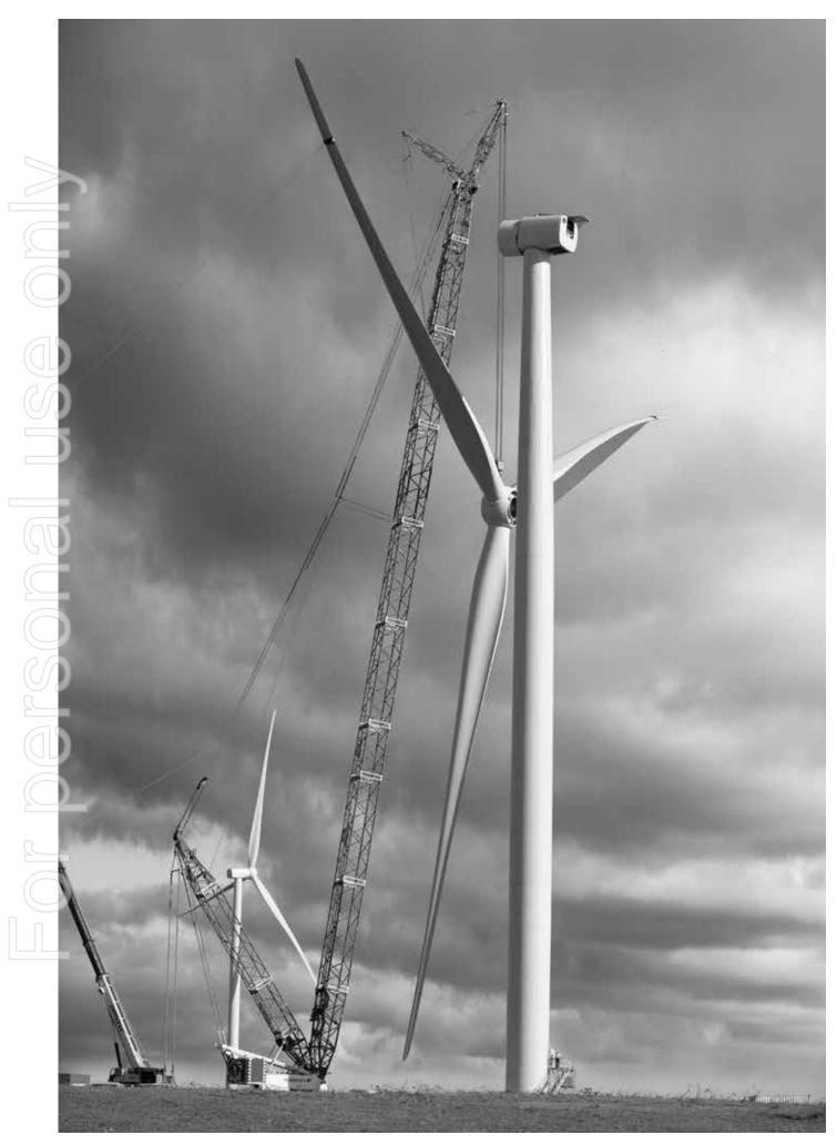
Erecting one of Waipipi Wind Farm's 31 turbines 7 kilometres southeast of Patea. The blade tip reaches 160 metres from the ground
