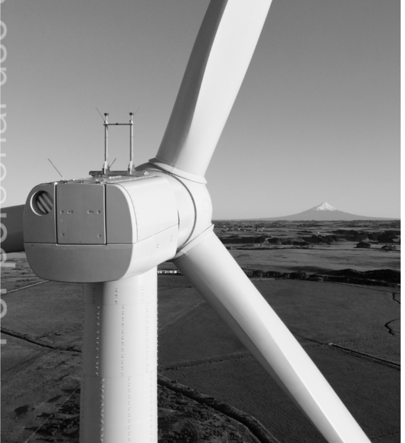
Waipipi Wind Farm's first turbine
