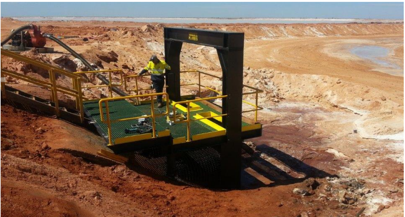
Figure 7.3. Typical Weir Platform Installation for Ponds
