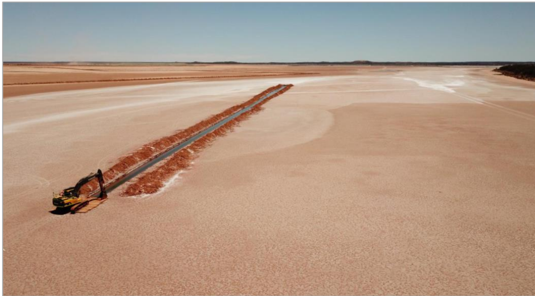
Figure 3.2: Trench Excavation (T Swierczuk, Feb 2020)
