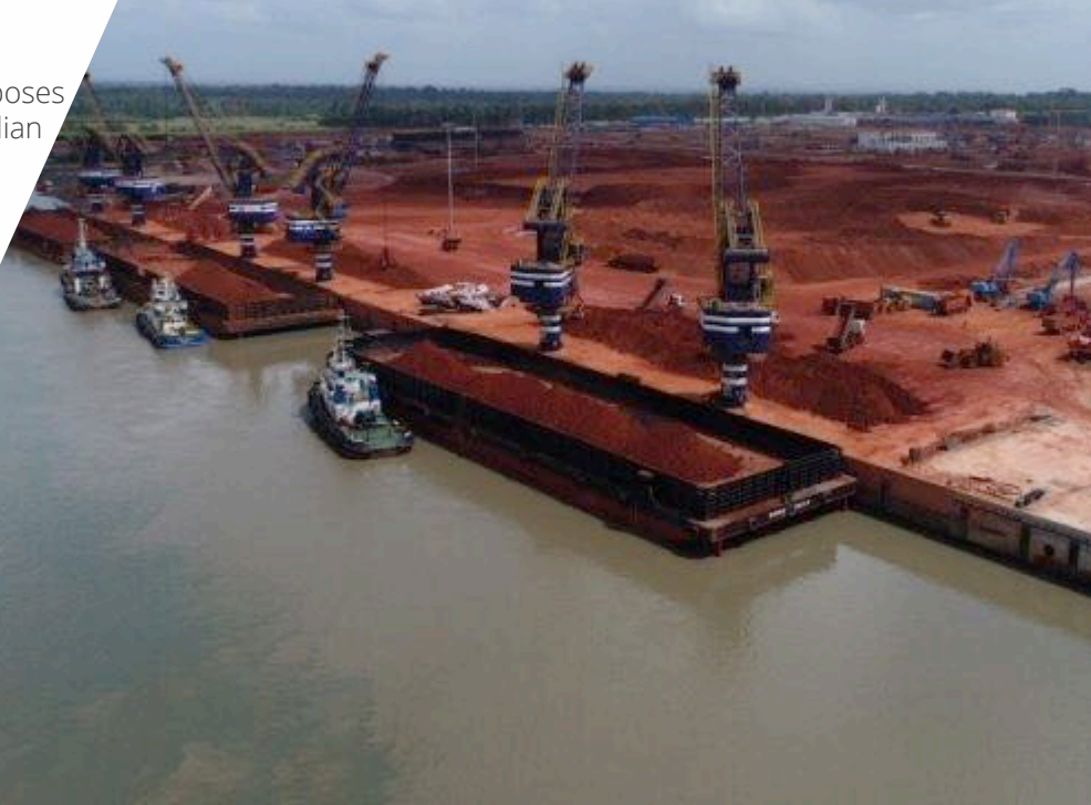
Image 1: SMB barge loading at Katougouma terminal
