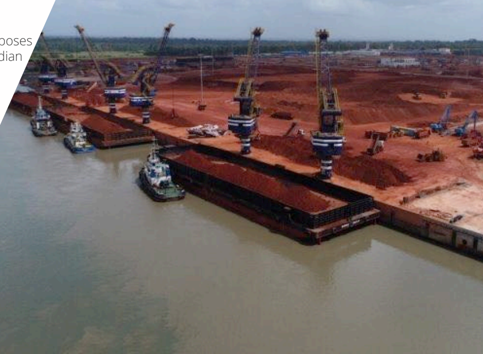
Image 1: SMB barge loading at Katougouma terminal
