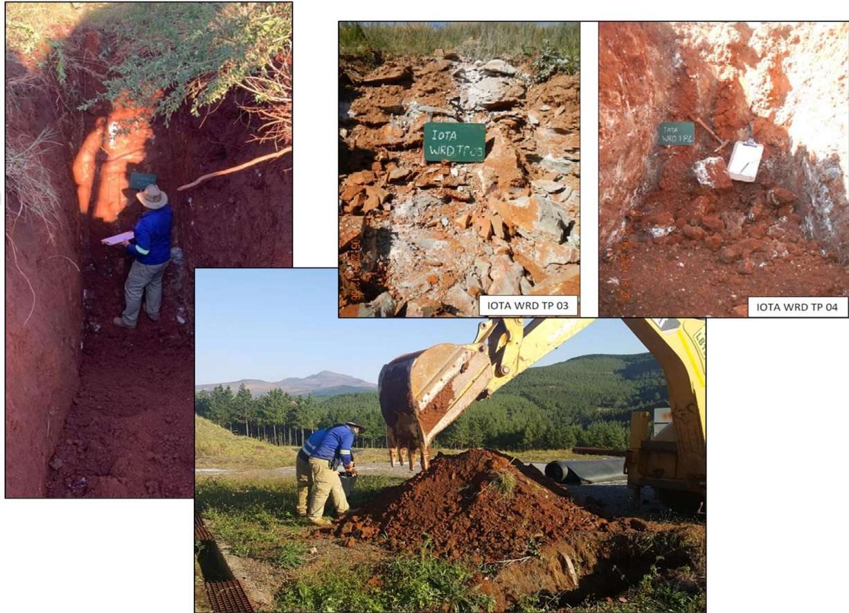
Figure 2: Test pits for ground stability
