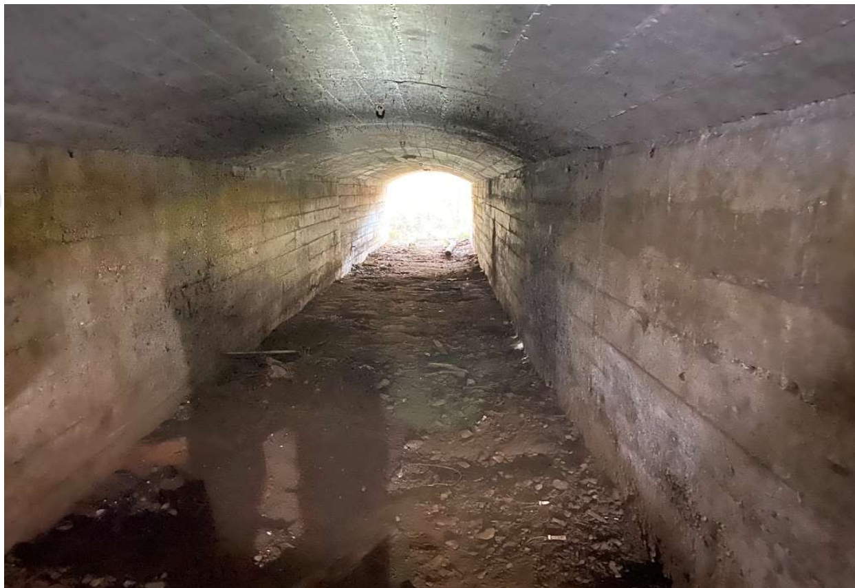
Figure 11: Clewer Dukes Morgons Mine Access Portal
