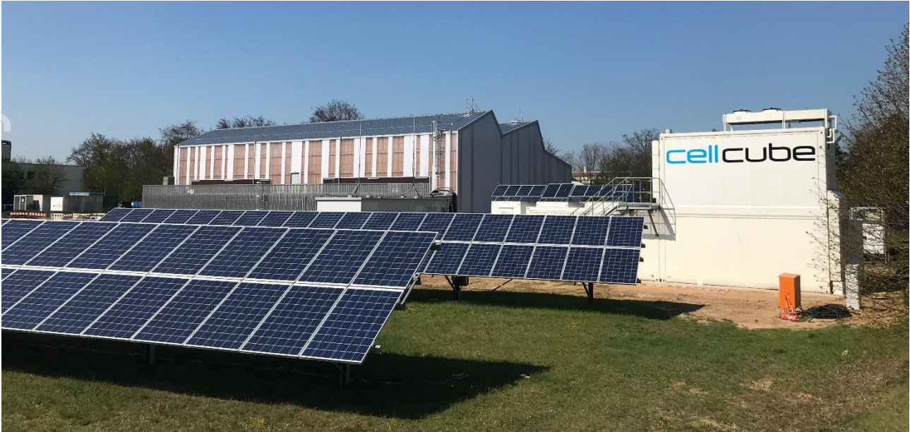
Figure 5 Solar and CellCube VRFB installation at a commercial and industrial site © Enerox
