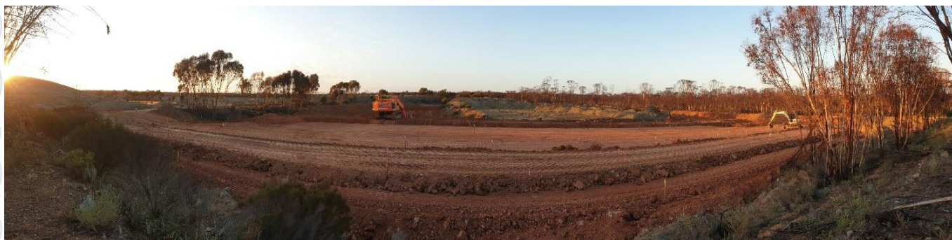
Heap leach pad construction
