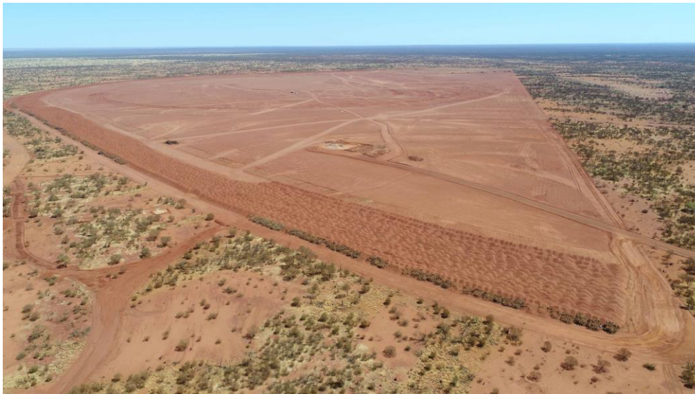
Clearing and topsoil removal for the TSF/IWL
