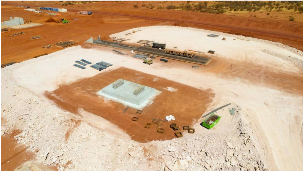
Fine ore stockpile and reclaim tunnel
