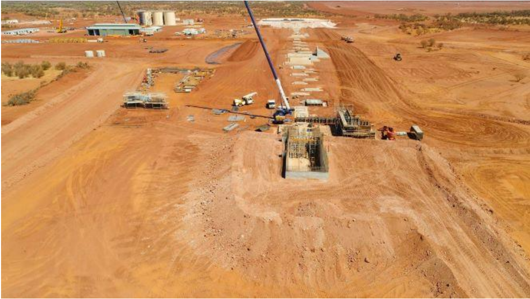
Foundations for crushing circuit
