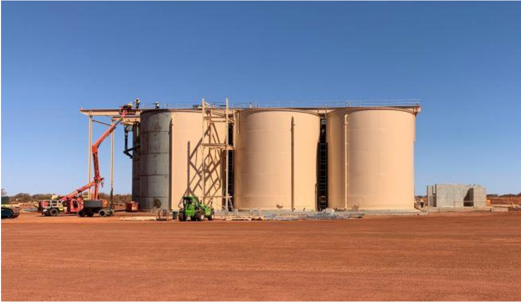
CIL tank steelwork and painting
