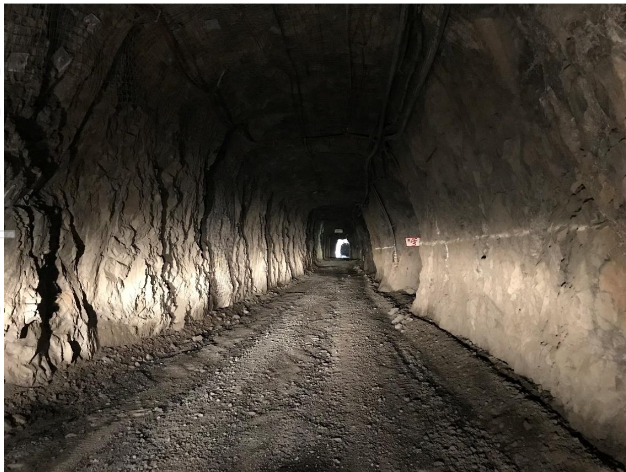
Figure 7 Metz Mining Centre Decline
