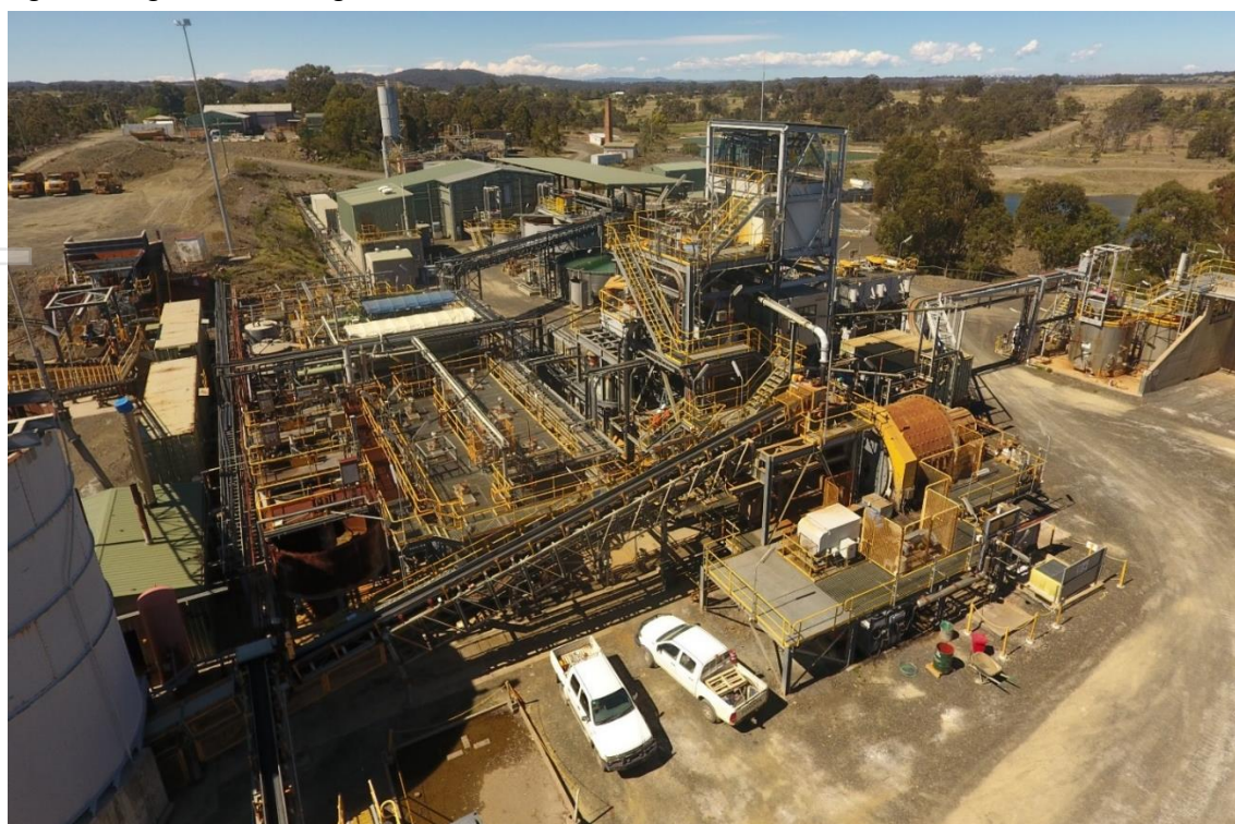
Figure 2 Hillgrove Processing Plant
