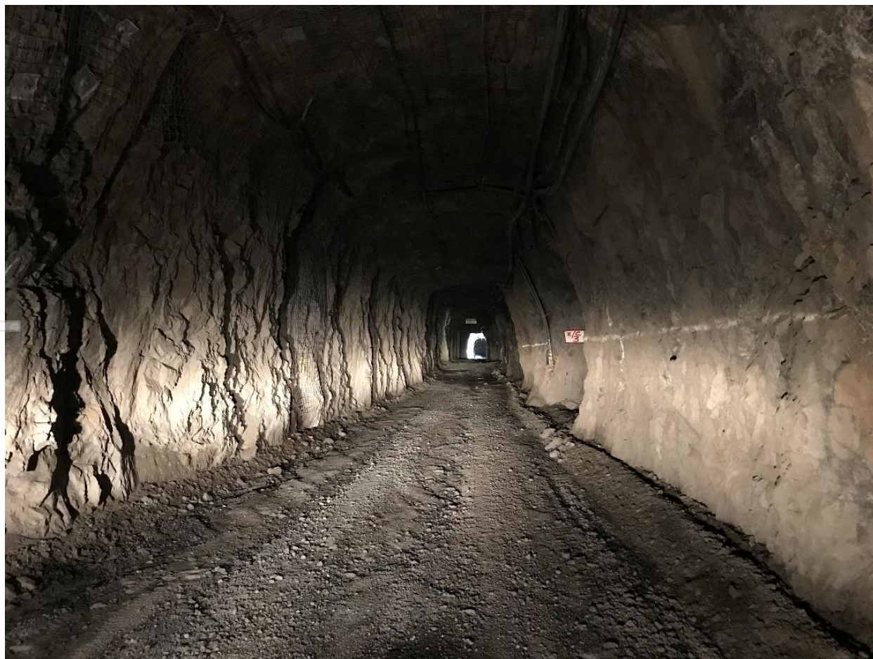
Figure 7 Metz Mining Centre Decline
