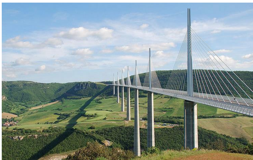
The addition of 0.0025% of Niobium to the steel in the Millau Viaduct reduced the weight of the steel and concrete by 60% in the overall project (Source: CBMM)
