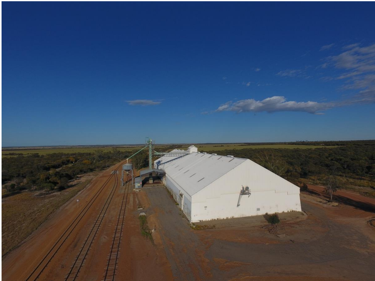
CBH Gabbin's storage shed, road and rail loading and siding facilities
