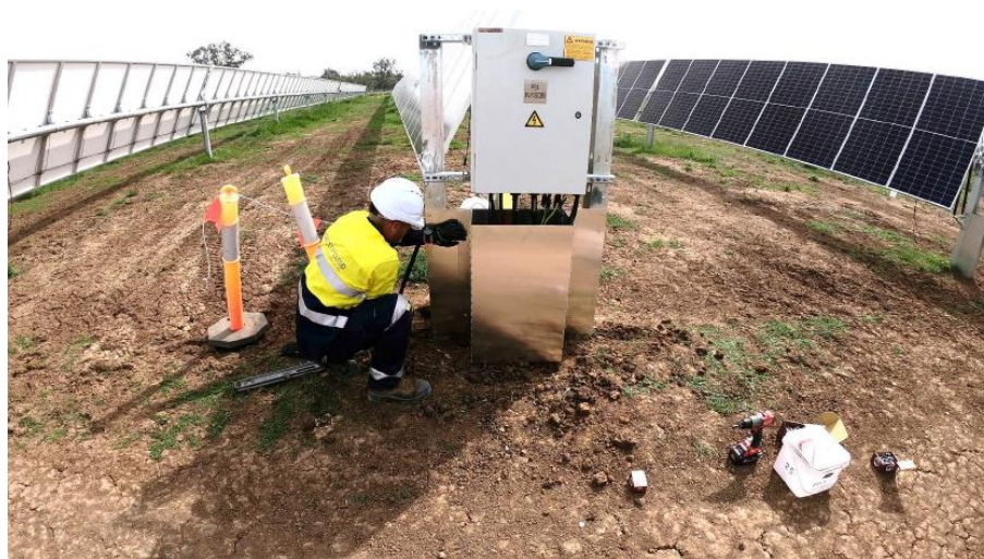
Figure 2. Jemalong Solar Project Panel Installation
