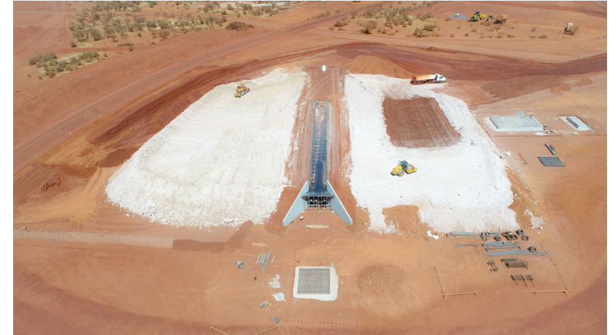
Fine ore stockpile preparation
