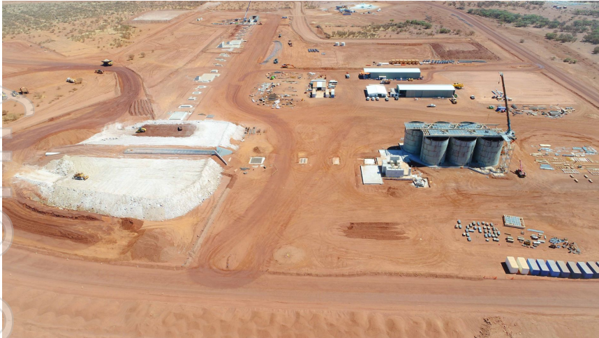
Process plant construction
