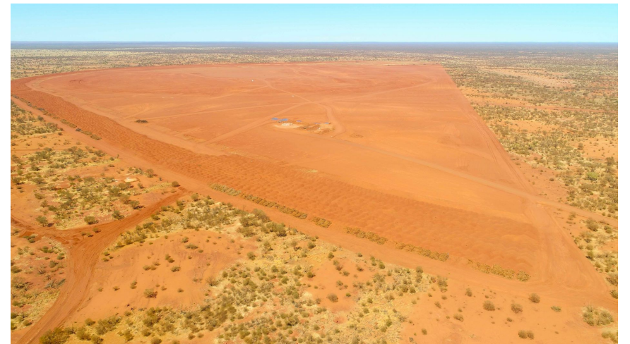
Clearing for TSF
