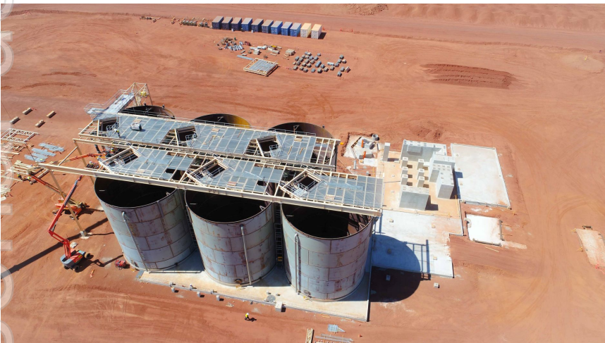
CIL tank erection
