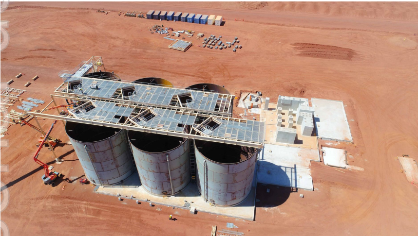
CIL tank erection
