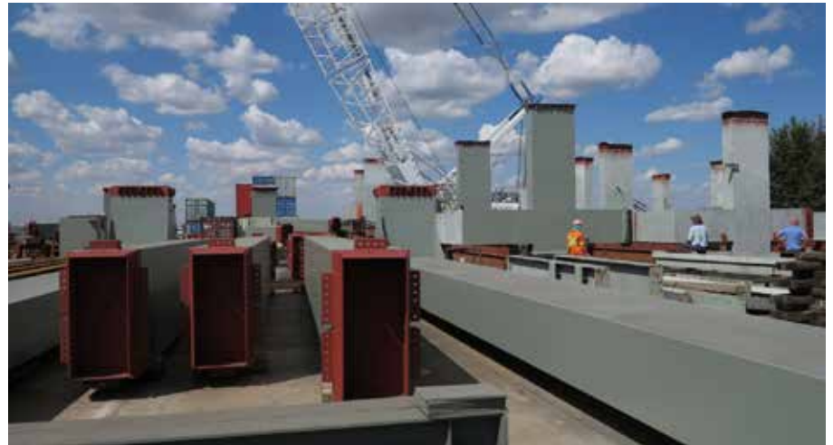
Headframe Structural Steel well advanced in its Refurbishment Program.
