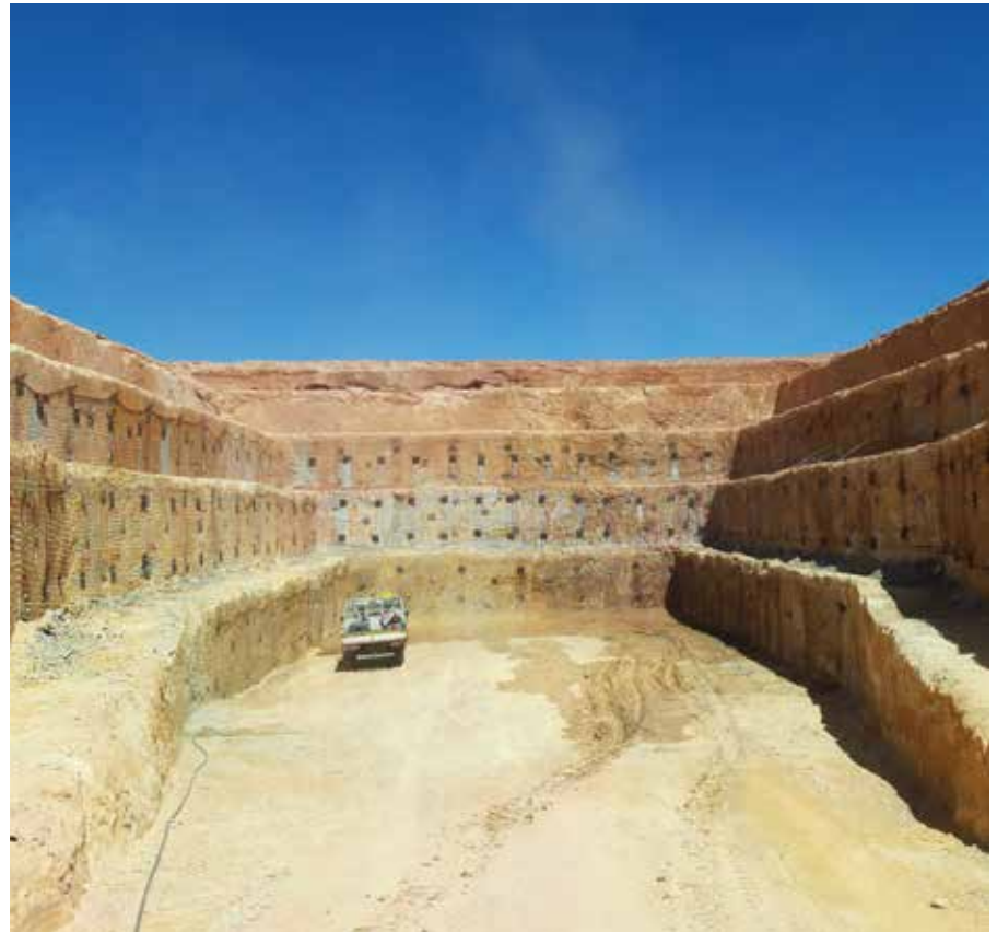
Completed box-cut for shaft collar civils.
