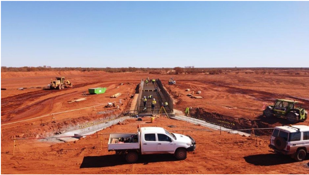
Fine ore stockpile tunnel concrete footing
