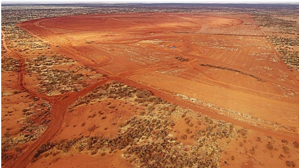
Clearing and topsoil removal for the TSF/IWL
