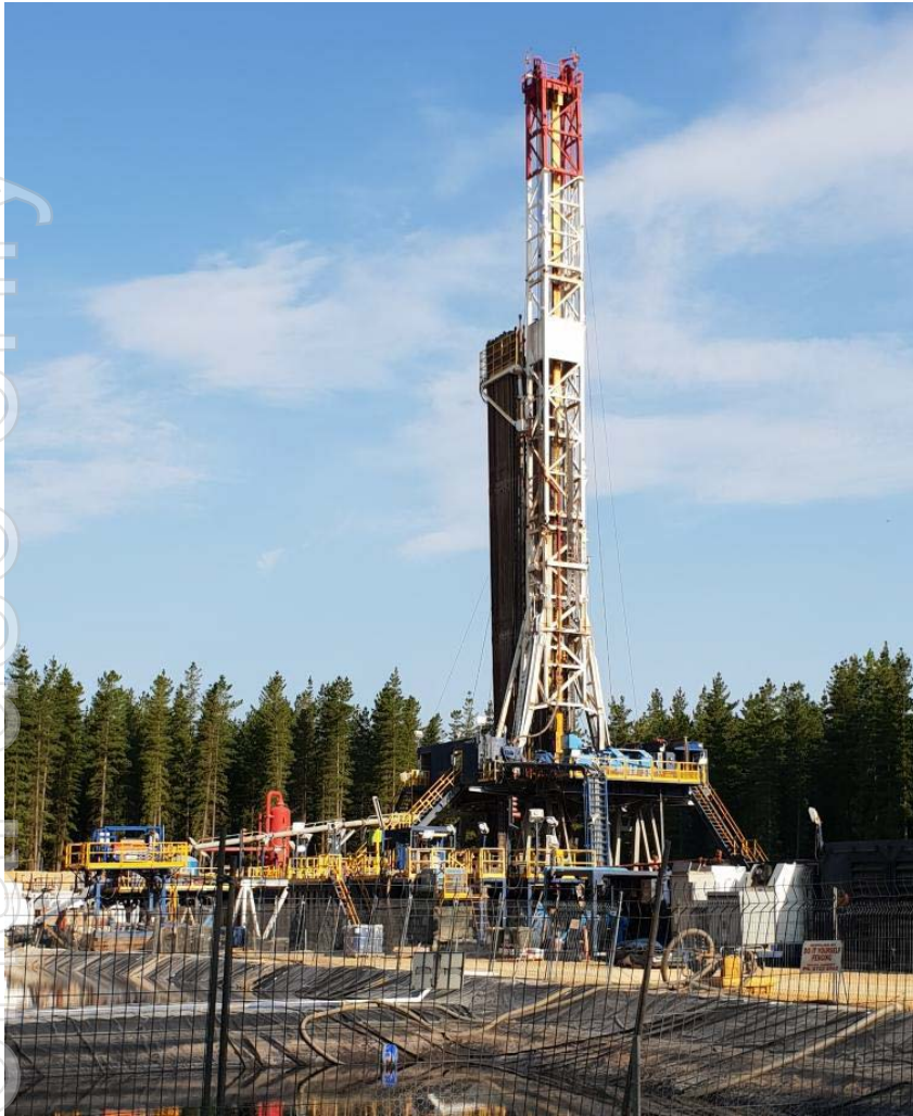
Easternwell Rig 106, on-site
