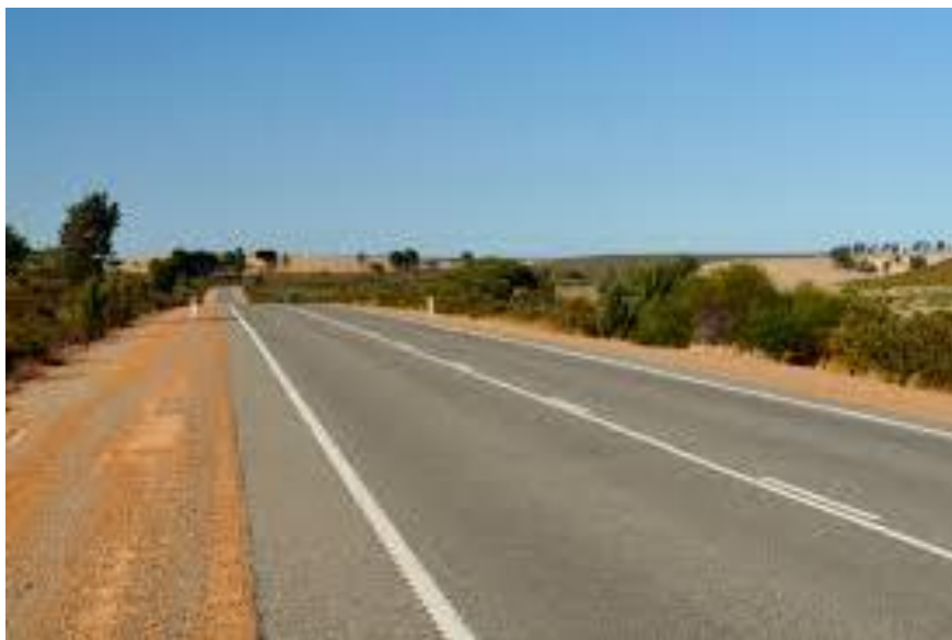
Brand Highway Proximal to Beharra
