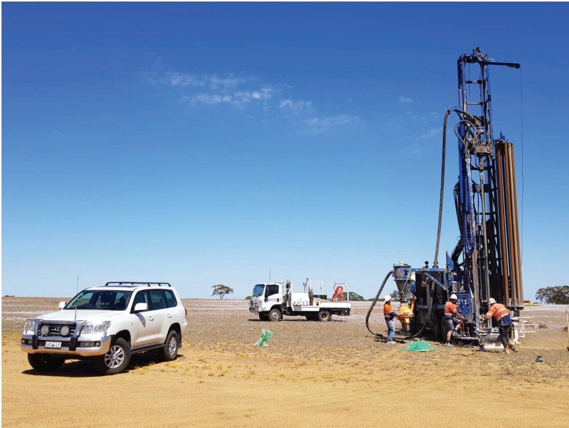
Figure 15 2019 Water Bore Air-core drilling program.
