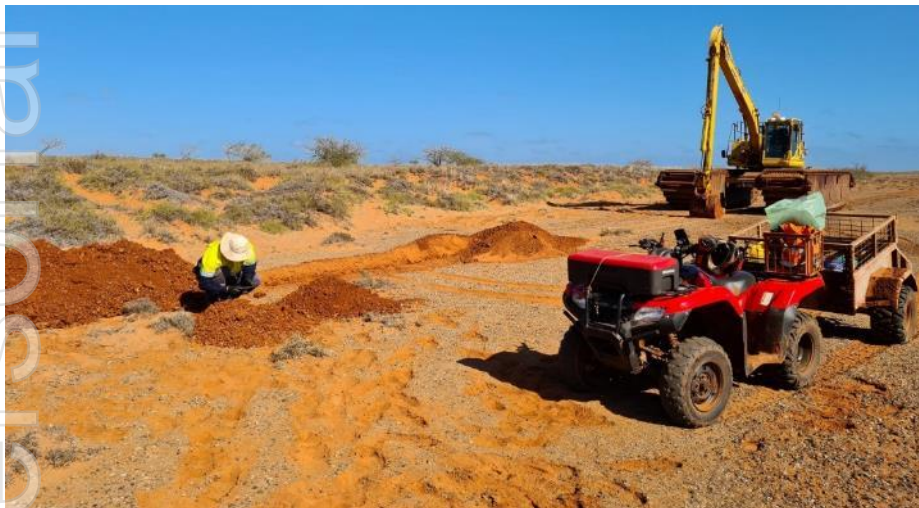
3. GEOTECHNICAL TEST PIT FOR FEED
